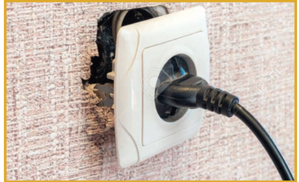
Damaged electrical sockets and wires
