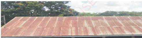
Figure 7.8: Rusted iron sheets
